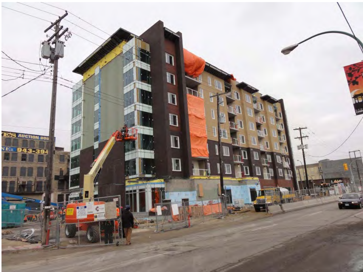
Peace Tower Housing Complex under construction
